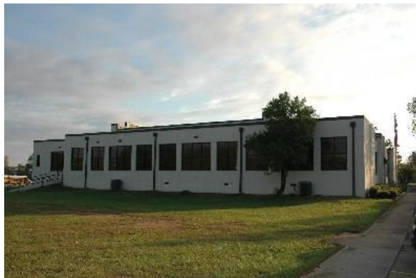
Willis ISD Cargill Education Center - Before!
